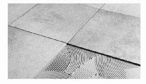
Build resilient and durable outdoor spaces, pathways, driveways, and more with the installation of 20mm tiles on screed with adhesive.
